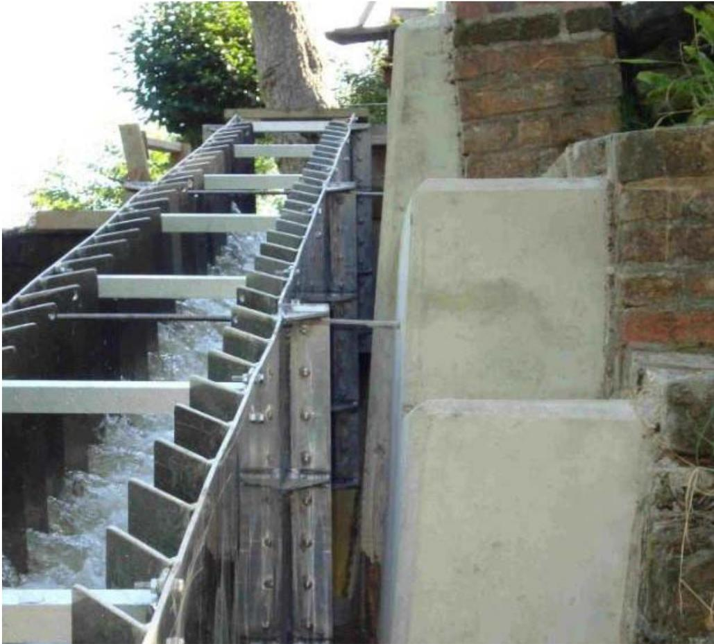
**Figure 2.1. A free-standing Alaskan fish pass, showing the metal baffles extending up each side of the pass.**
