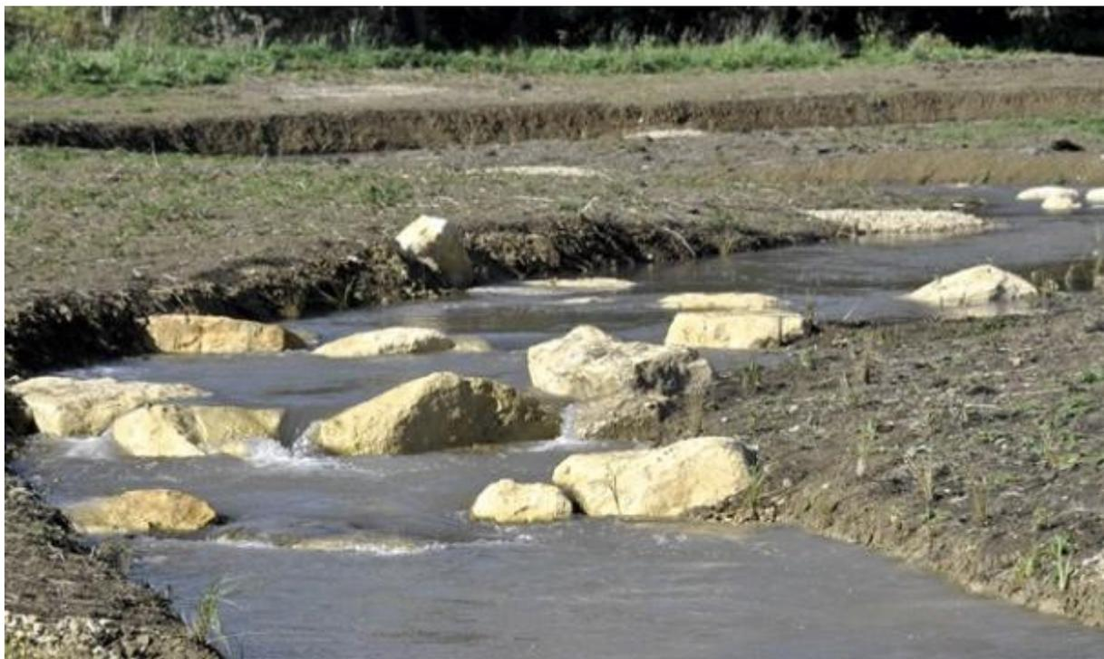
**Figure 2.5. An example of a bypass channel set at a slope of 5 %. Boulders have been added to the channel to reduce mean water velocities.**
