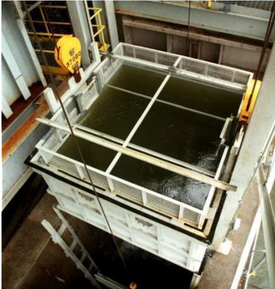
**Figure 2.3. An example of a fish lift used to transfer American shad upstream of Holtwood Dam on the Susquehanna River, USA.**
