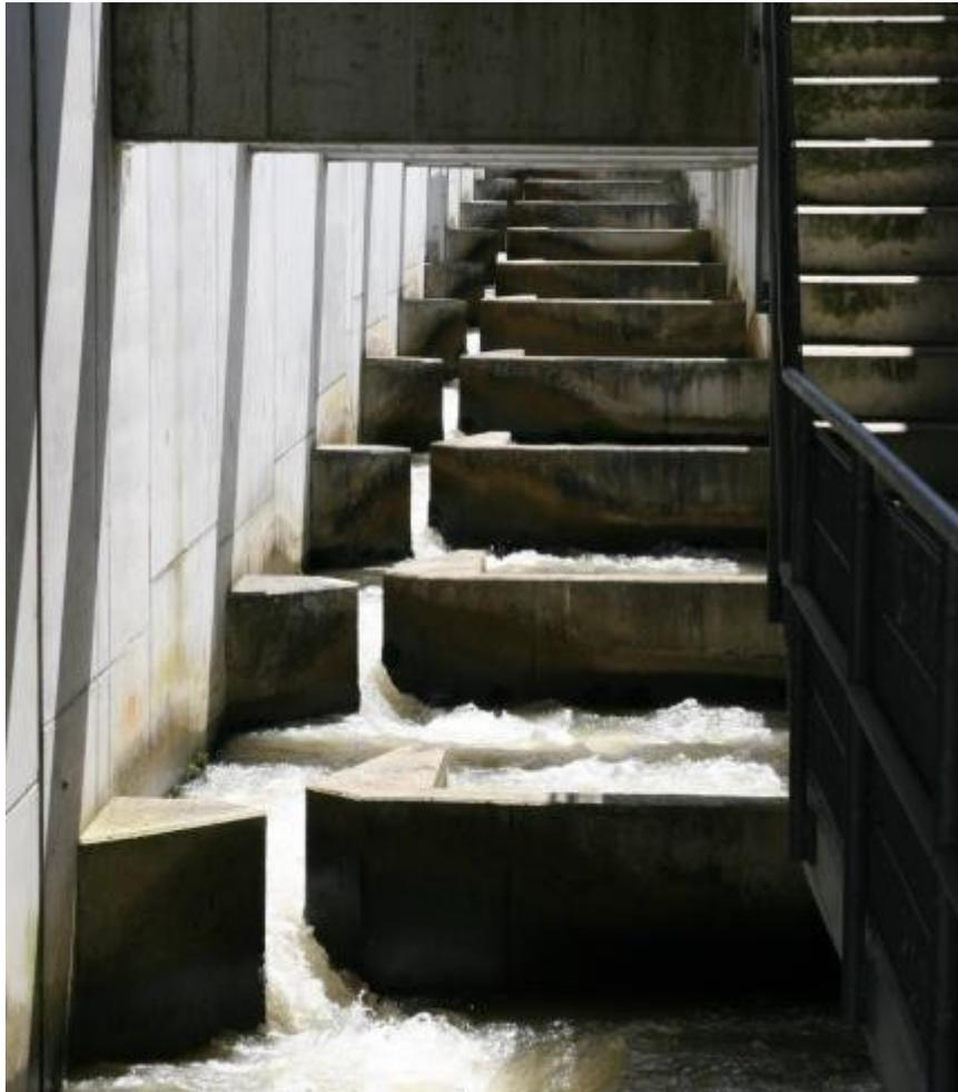
**Figure 2.4.** An example of a large vertical slot fish pass on the River Rhine that facilitates the passage of allis shad upstream of the 10 metre high Iffezheim Dam.
