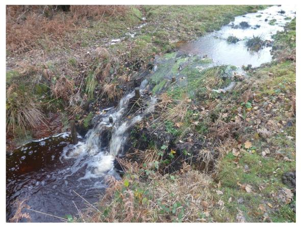
Figure 1-10: Infilled staked bales to raise water levels
