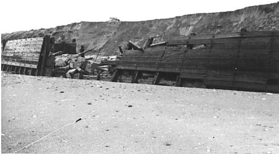
**Figure 18 January 1960: Collapsed revetment along the Neck (from Phillips 1962)**
