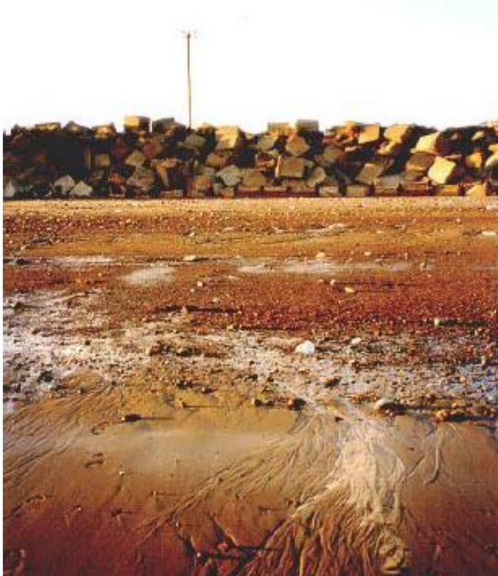
**Figure 23 1997: Concrete block seawall/revetment along the southern part of the Neck (from Nicholas 2003)**
