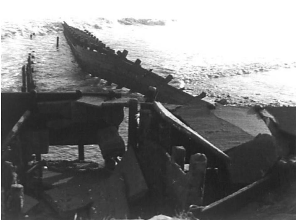
**Figure 20 January 1960: collapsed revetment along the Neck – it appears to be fronted by a timber framework and topped with thin concrete slabs (from Phillips 1962)**
