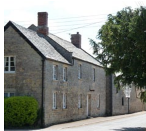
Simple vernacular architecture using local 'blue' Lias limestone in the burtle village of Chedzoy.
