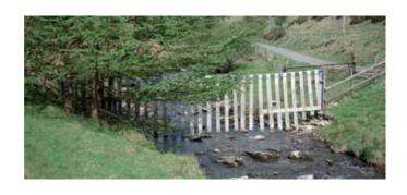
river or stream flood and the gate be destroyed then the main fence will remain undamaged.
