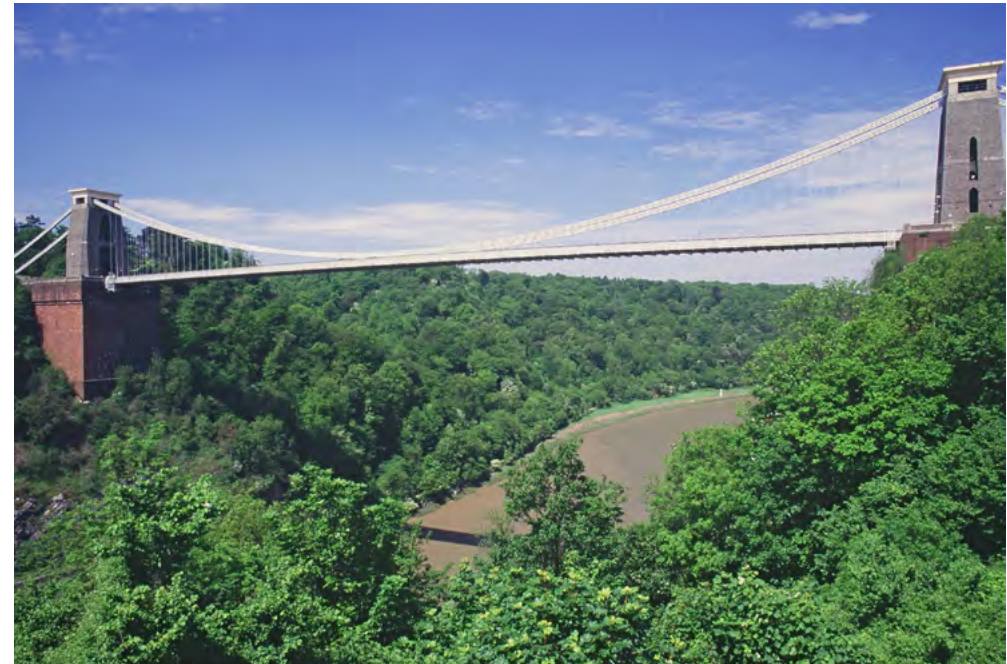
The Clifton Suspension Bridge rising above the Avon Gorge, designed by Isambard Kingdom Brunel but constructed after his death.
