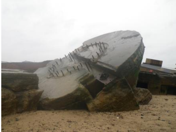
Photo 14 The mounting for the southern 9.2 inch gun; it is surrounded by pieces of the concrete apron
