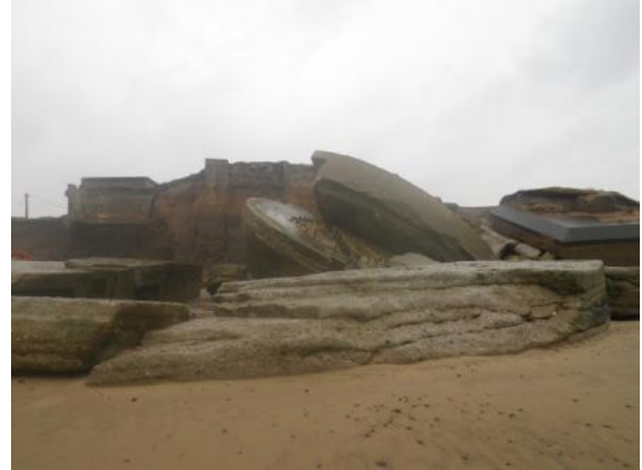
Photo 17 The apron and mounting for the northern 9.2 inch gun (the magazine is on the right)
