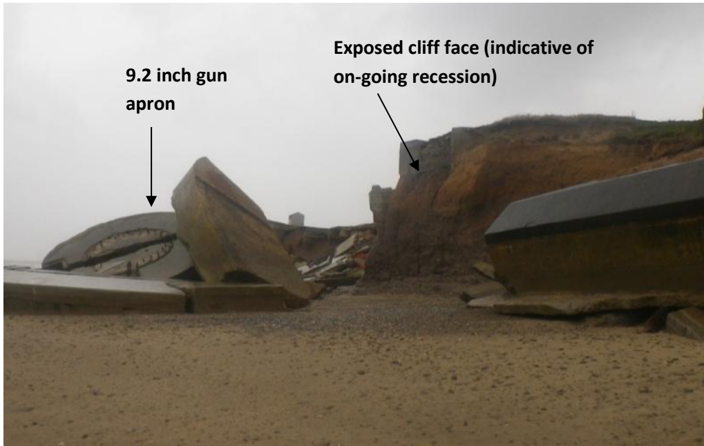
Photo 20 Exposed cliff face behind the northern 9.2 inch gun apron
