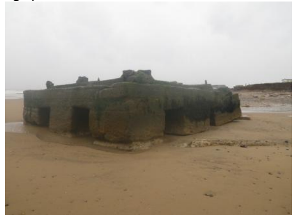
Photo 18 Remains of a concrete building (possibly the southern BOP blockhouse)
