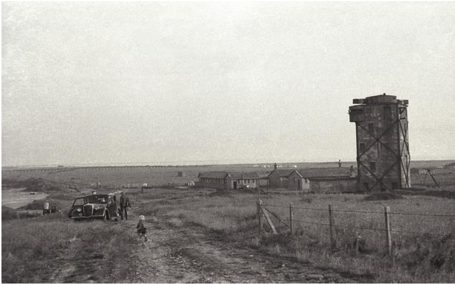
Photo 5 Godwin Battery southern battery observation post (the tower on the right), around 1958, showing the open ground in front of the site (source: http://www.derelictplaces.co.uk/main/showthread.php?t=20558 )
