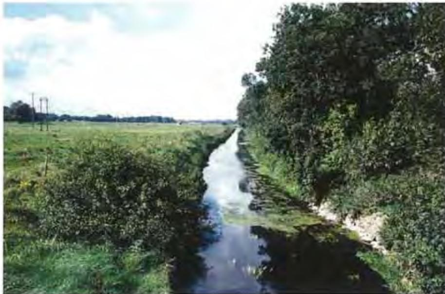
Plate 23 Resectioning on the River Lark, leaving a straightened and over-deep channel with greatly reduced habitat diversity
