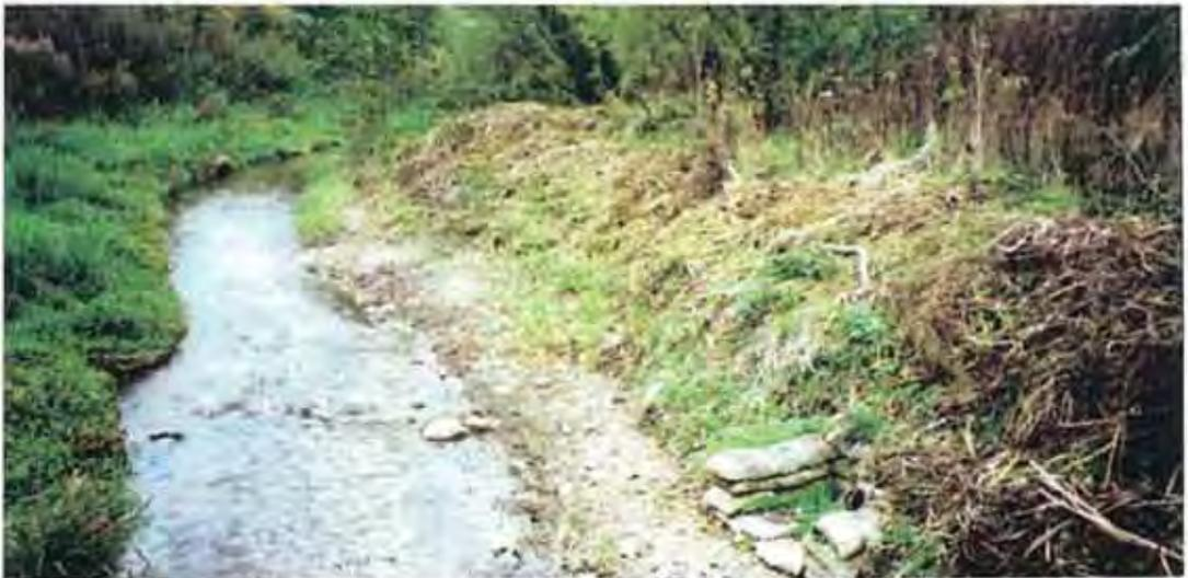
Plate 36 The same section of the Misbourne following limited removal of plants and silt across half the width of the channel (29 September 1994).
