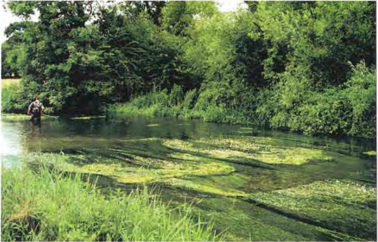
Plate 34 Weed cutting to leave strips of vegetation across the channel so that water levels are maintained.
