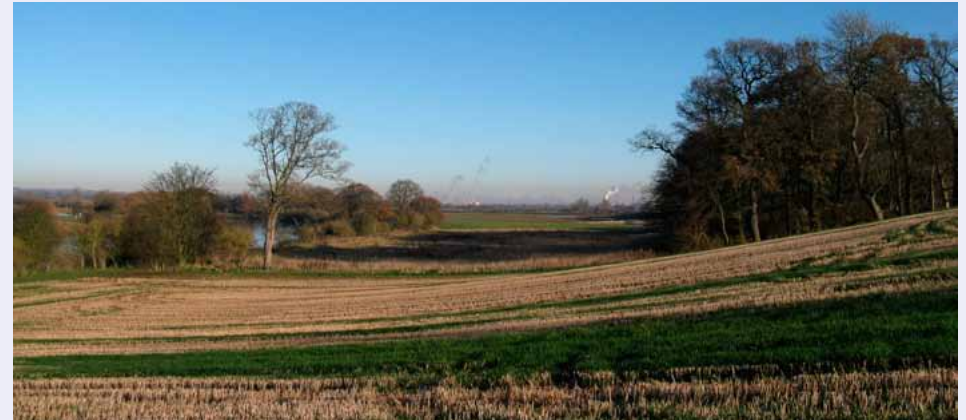
Some of the key characteristics are displayed in this view near East Stoke: arable farmland, the meandering River Trent, gently undulating topography. The plumes in the distance rise from Staythorpe gas fired power station and Newark sugar beet factory.
