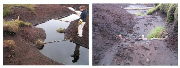
Figure 3-36: Infilling a gulley with vegetation after the installation of plastic sheet piling (from Evans et al., 2005)
