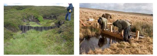
Figure 3-32: Plastic Sheet Pile Dam (left) and Wooden Pile Dam (right) (from Evans et al., 2005 and http://www.exmoornationalpark.gov.uk/wetland\_award\_project\_final\_report.pdf)
