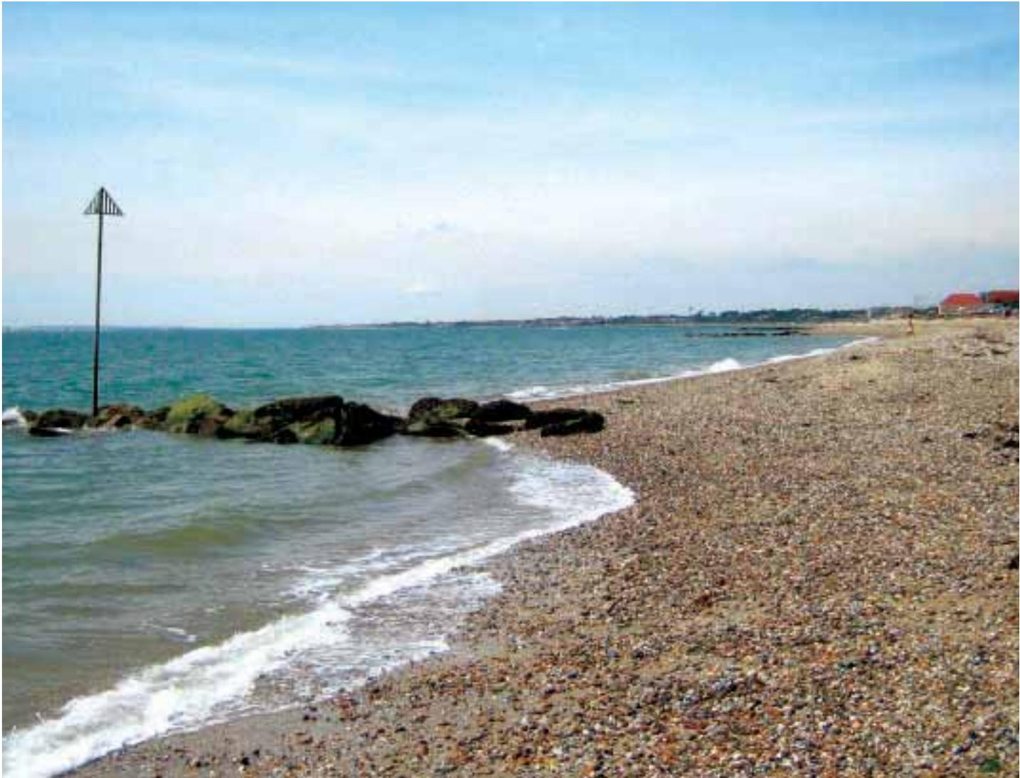
Replenished shingle material and rock groynes at Lee-on-the-Solent. Fine sediments imported with the shingle were selectively transported offshore and deposited as a thick drape over the interest features.
