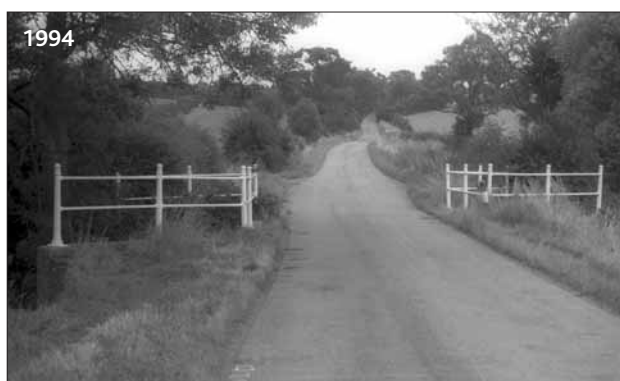
Figure 103: Traditional iron railings (top) have been replaced by standardized steel components at every stream crossing in the Huntingdonshire study area, identical at two different locations in 2005.
