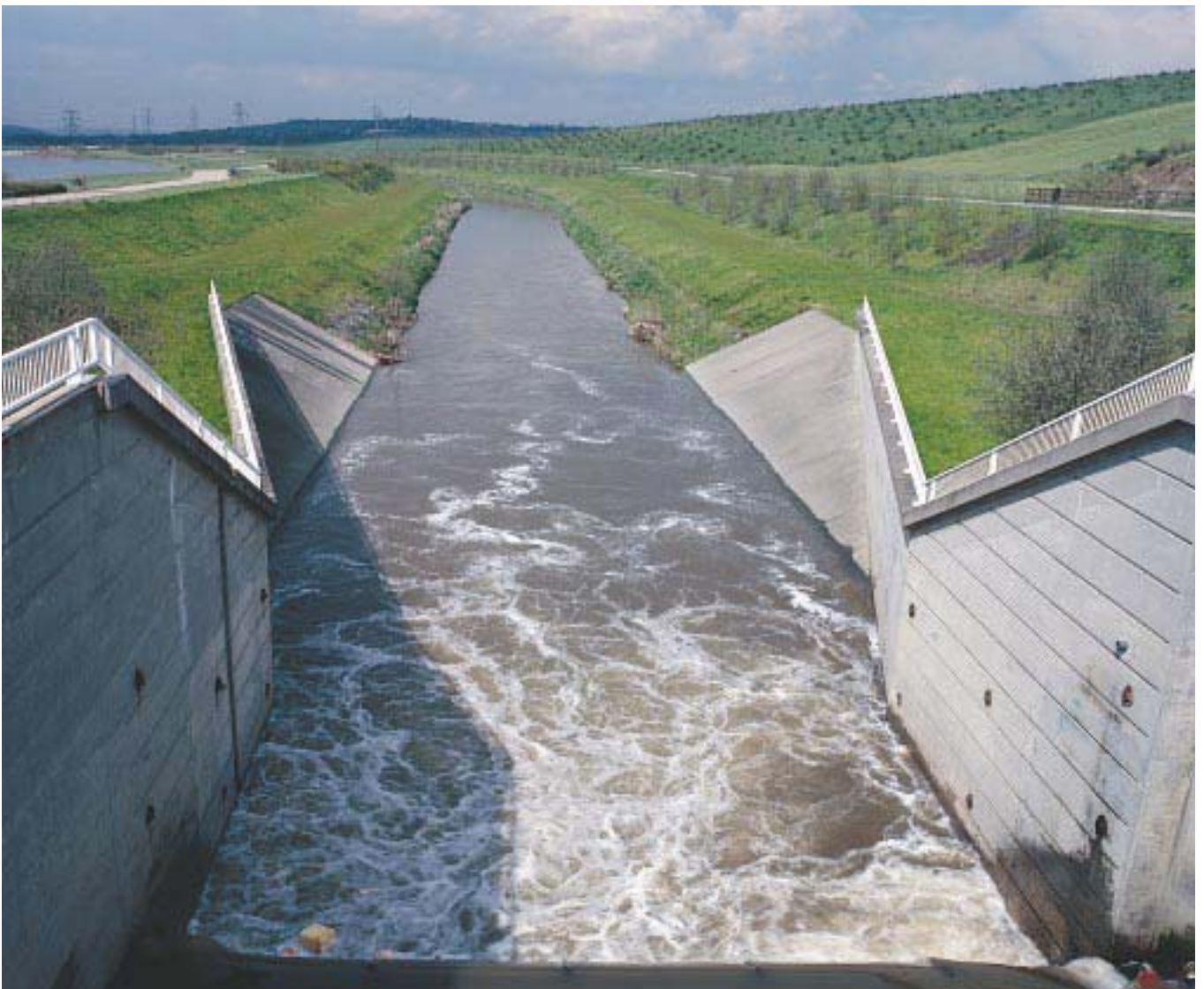
Confining rivers to fixed channels speeds the passage of water - River Rother. Peter Wakely/English Nature 8,183
