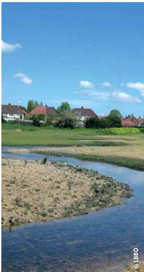
Creation of 500m of new sinuous water channels help to slow high flows and improve habitat diversity
