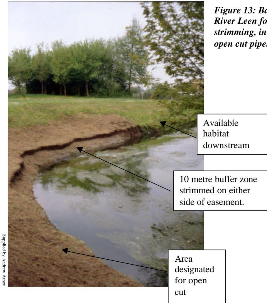
**Figure 13: Banks of the River Leen following strimming, in advance of an open cut pipeline crossing**
