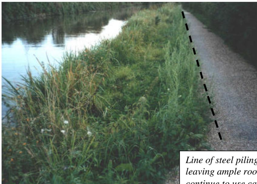
*Line of steel piling set under towpath, leaving ample room for water voles to continue to use canal banks*
