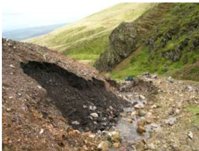
A diverted stream has caused erosion of the mine spoil dump. © Hannah Townley
