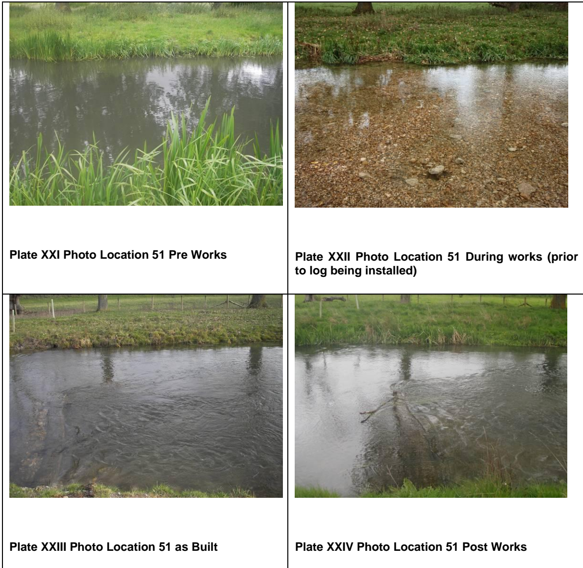
Figure 5.4 Log Deflectors in Reach 4 at Photo Location 51
