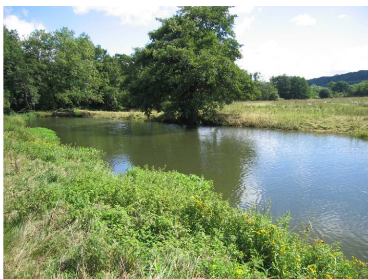
Photo FOR01s: Looking across downstream towards iron hatches structure at the downstream site boundary.
