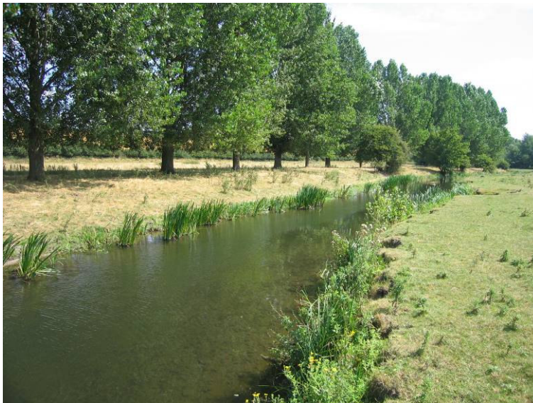
Photo SHR02f: Looking downstream along uniform glide section downstream of the Seven Hatches structure.
