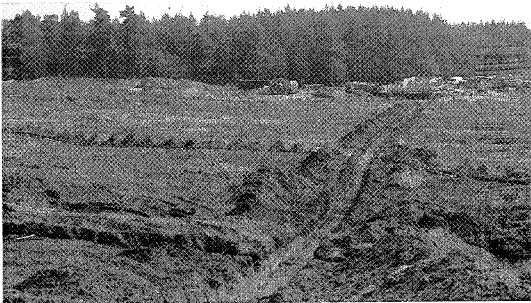
Plate 2. Habitat creation planning - use of field trial information. The results of the field trials at Cove Radio Station, Farnborough, were put into practice during the construction of the radio station. The results guided the creation of soil profiles, nutrient and pH adjustments, and the seeding prescriptions used in the restoration. September, 1990.
