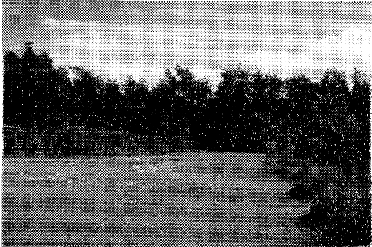
Plate 3. Ecoduct at Boerskotten (east of Oldenzaal): showing vegetated area on top of ecoduct (note high sides used to screen large animals from noise and lights of traffic below)
