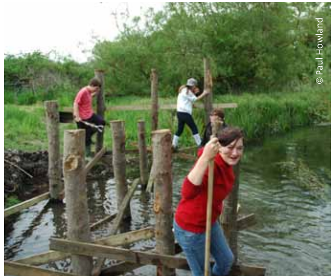
Young people building a river dipping platform on a farm
