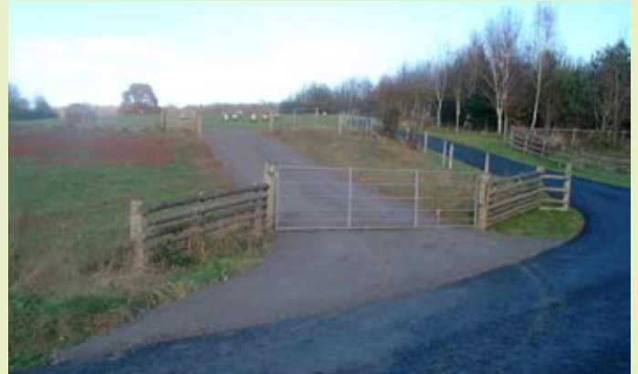
Access track and gateway after ECSFDI grant work
