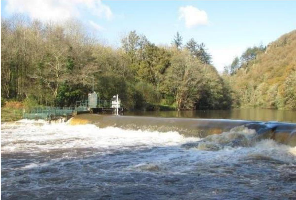
**Figure 1.8. A photograph of Gunnislake Weir facing upstream, showing the Cornish fish pass (left) and the Devon fish pass (right).**
