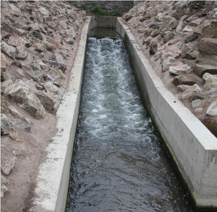
Figure 2.2. A Larinier super-active baffle pass showing the turbulent flow through the pass.
