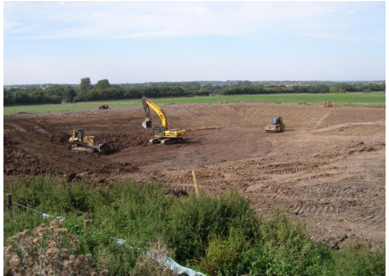
New earth banked lagoon being created
