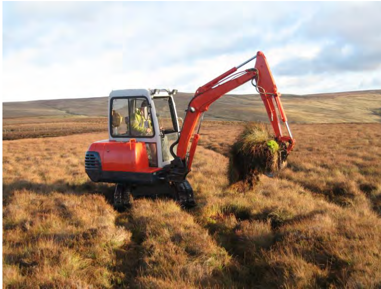
Photograph 6: Grip blocking being undertaken on Williamston as part of the HLS agreement.
