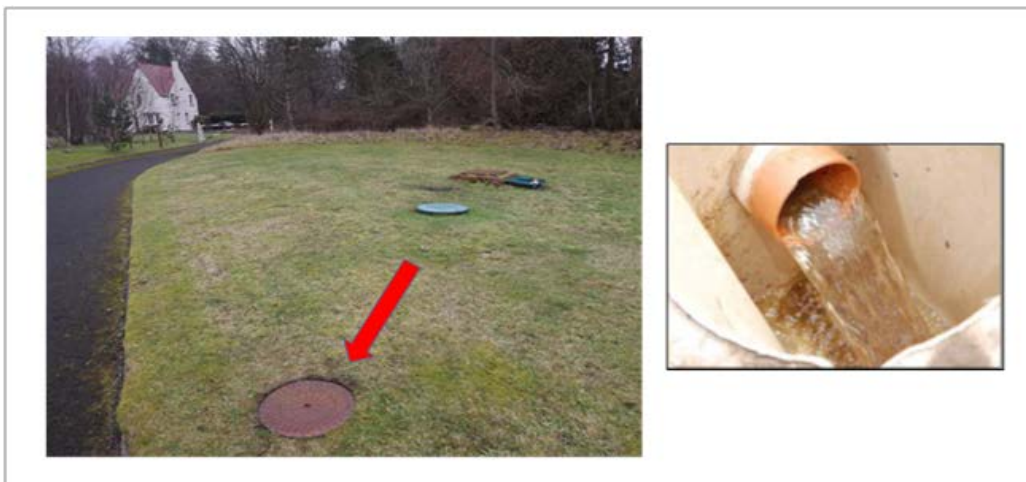
Plate 1 Location and sampling point for Tank 1, showing inspection cover and effluent sampling point within the inspection chamber
