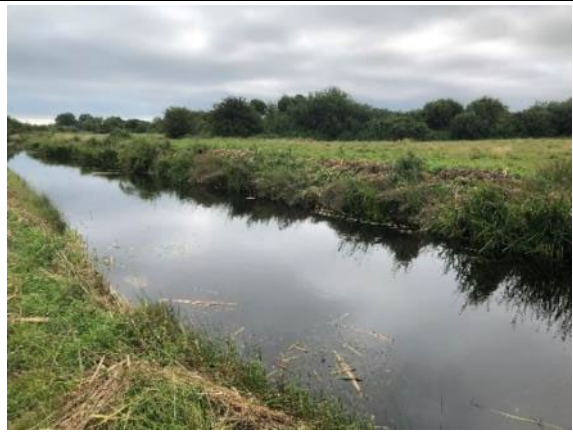
Main Down Sewer
