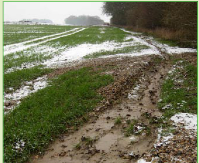
Material washed out by channelled water
