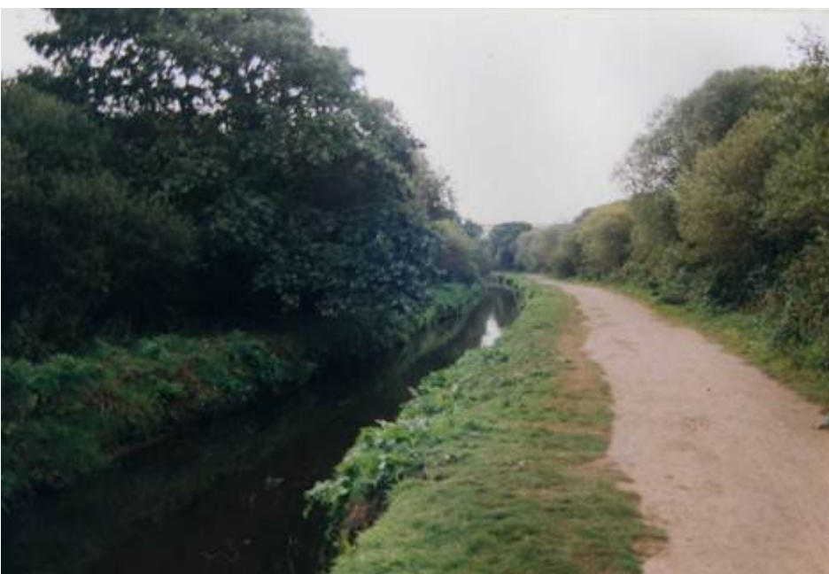
Figure 2.18 Channel straightening and bank reprofiling eliminating the natural river habitat mosaic
