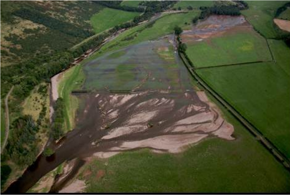
Figure 2.21 Channel avulsion caused by the pinning and embankment of the channel against the valley side to facilitate agricultural management of the floodplain (photograph supplied by the Environment Agency)
