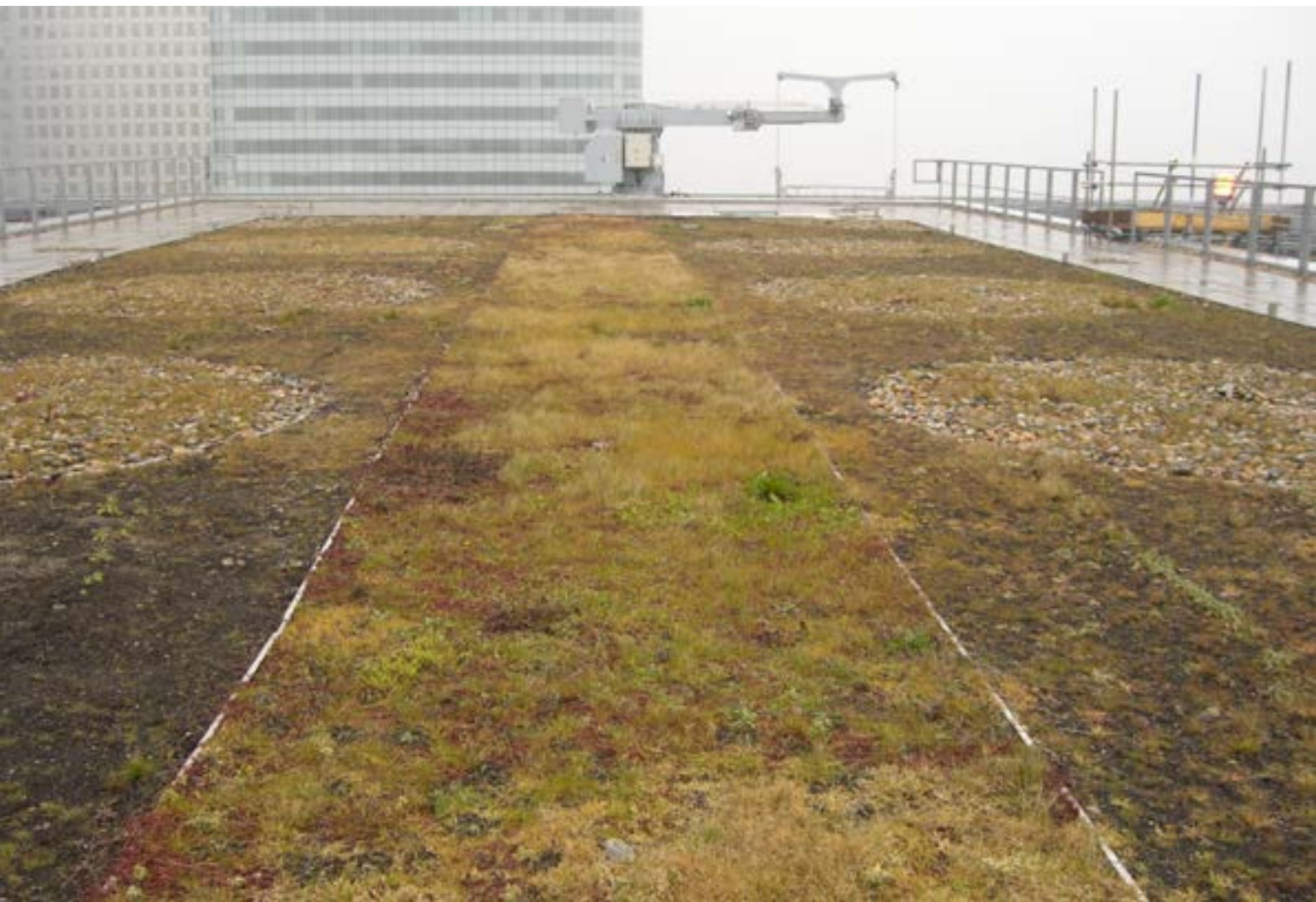
Green roof at Canary Wharf, London. © Natural England/Sarah Taylor
