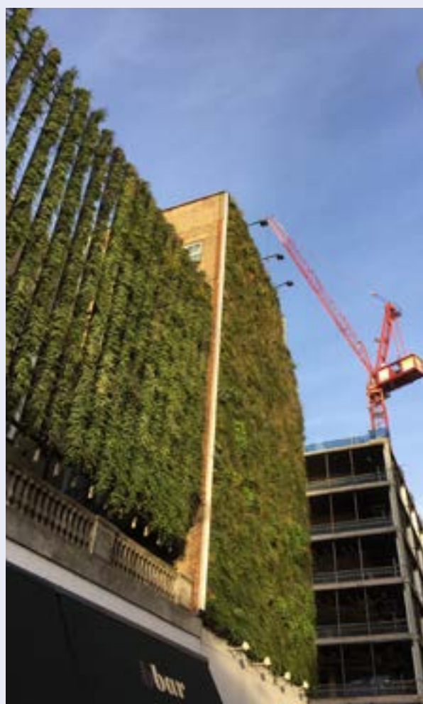
Retro-fitted green wall on the Rubens Hotel in Victoria. © Natural England/Sarah Taylor
