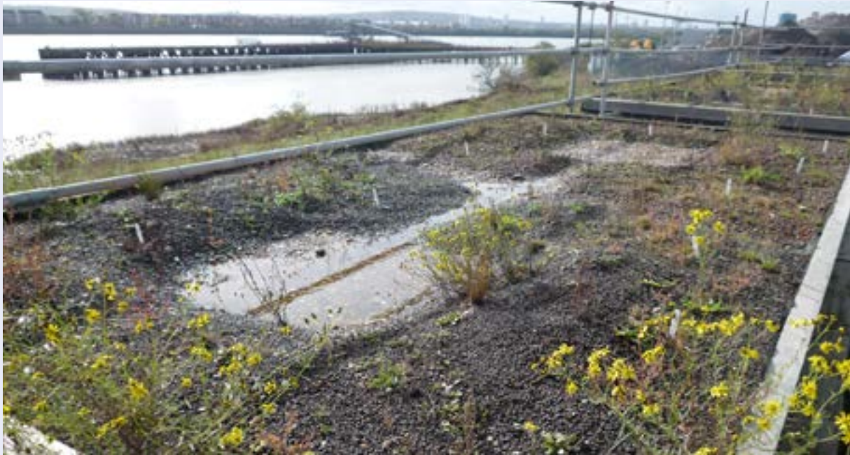
Wetland habitats created on green roofs. © Caroline Nash
