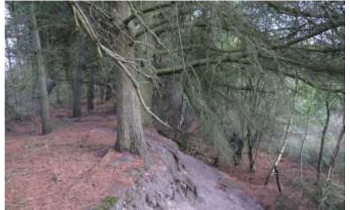
Four Ashes Pit SSSI before clearance. The former pit faces are heavily wooded which is preventing access to the geological profile.
