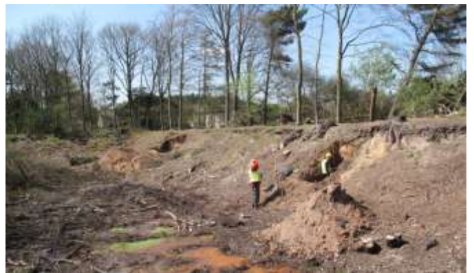
Four Ashes Pit SSSI after clearance works. Note the waterlogging in the former pit floor - here brash from the vegetation clearance was laid down to improve access.
