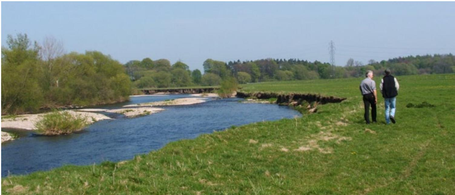
**River Swale at Great Langton:** The floodbank has been set back from the river here, creating temporary flood storage, wet grassland and natural features such as shingle banks, and allowing the river to meander in its floodplain.
