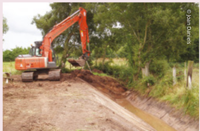
Deepening a ditch as part of project to divert enriched polluted water away from the core of the SAC.
