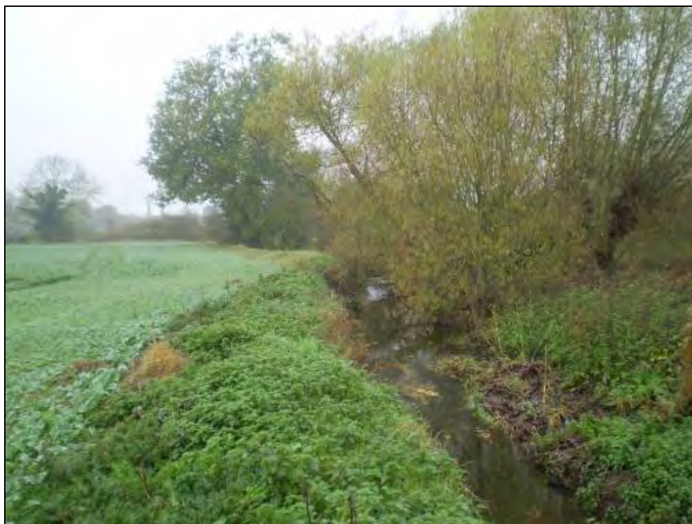
Figure 5.7: Low informal embankment along a section of Gilwiskaw Brook in reach GIL006
