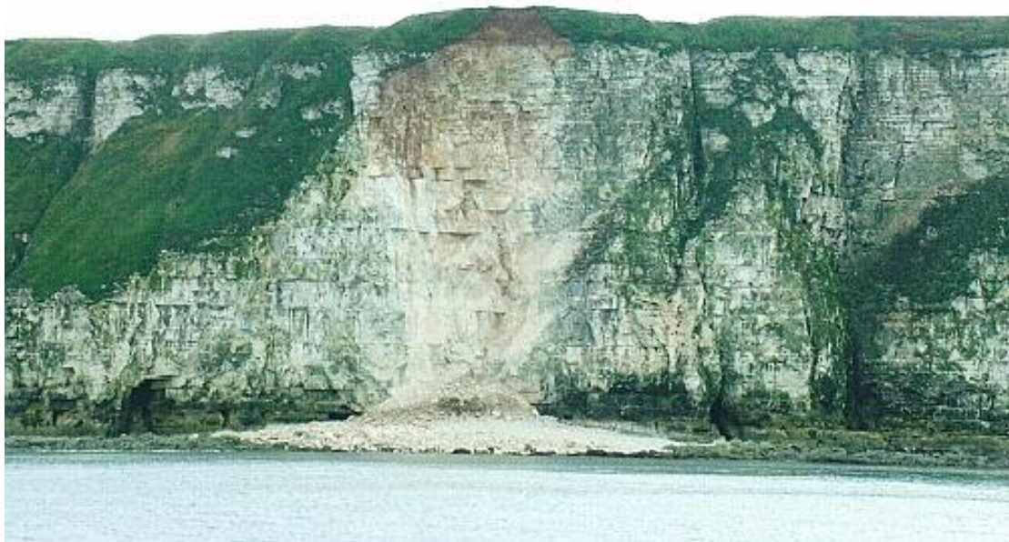
Figure 44: Rockfall on the Bempton cliffs - this occurred less than a week before the photograph was taken
