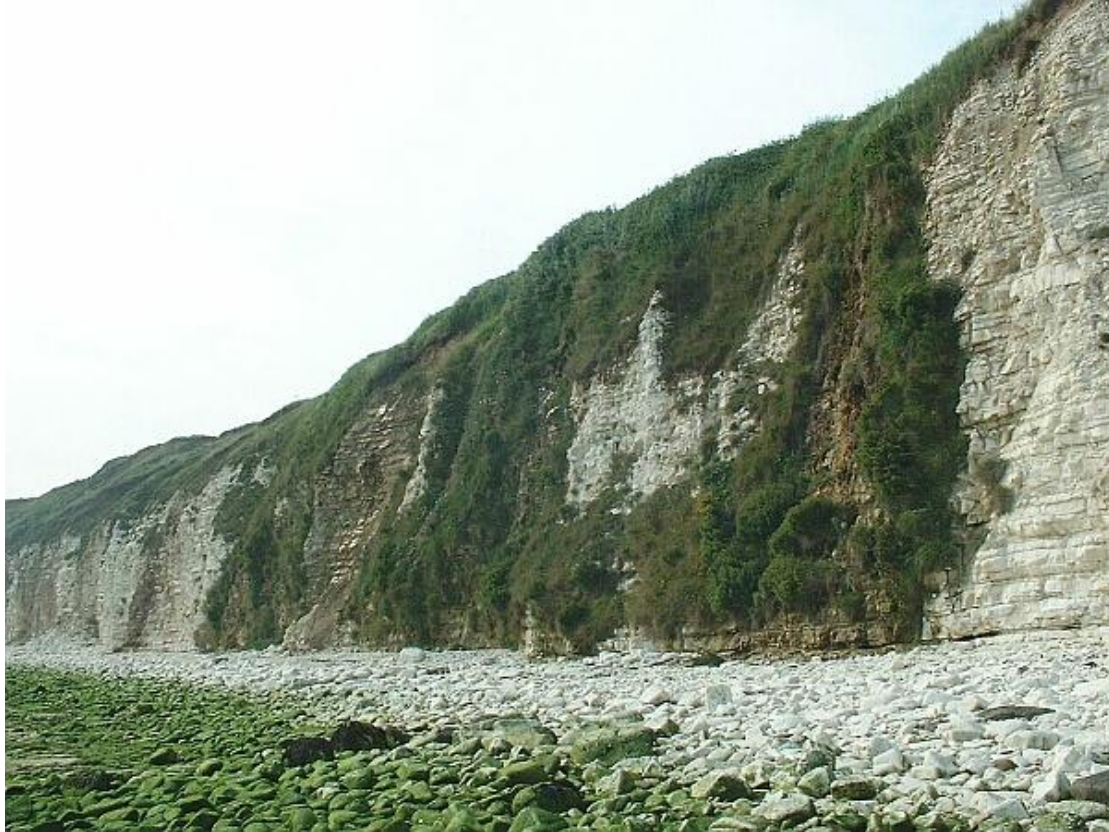
Figure 36: Flush vegetation on cliffs below Beacon Hill
