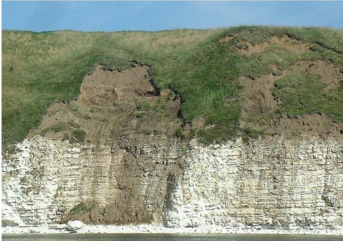
Figure 43: Collapsing upper (soft) cliffs to the east of South Landing
