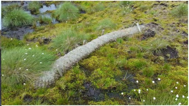
Fig. 6: Coir roll in amongst heather brash used to slow water movement across the bare peat surface.
