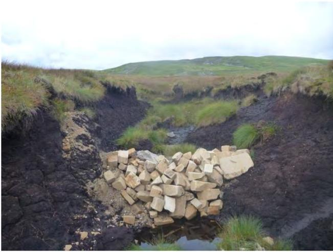
Fig. 5: Stone dam used as a sediment trap.
