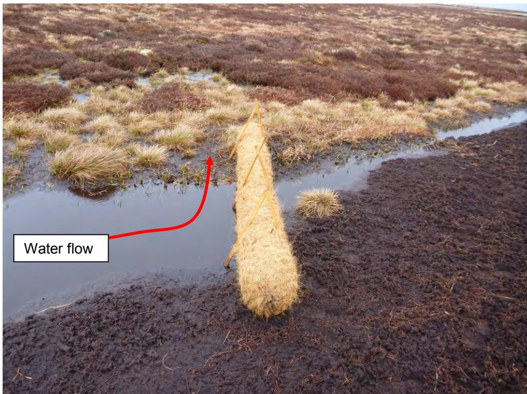
Fig. 2: Coir roll secured into place to divert water into existing vegetation
