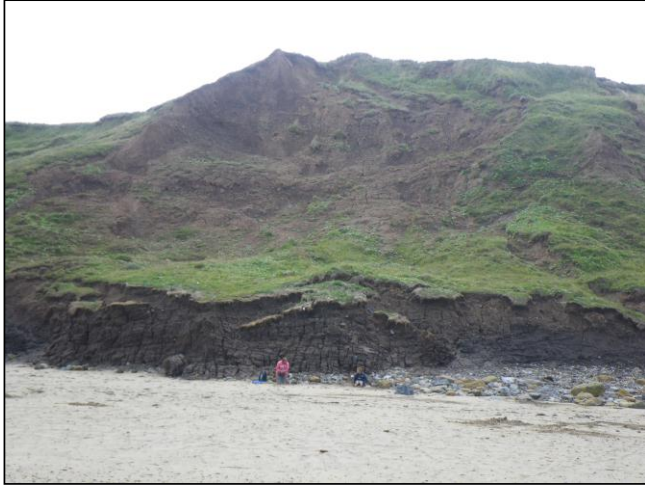
Photograph 25 Soft maritime cliff/slope with recent landslide. Severe wave erosion at base of slope.
