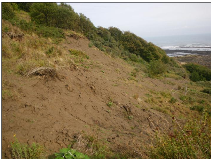
Photograph 81 Landslip with solifluction, Unit 1.
