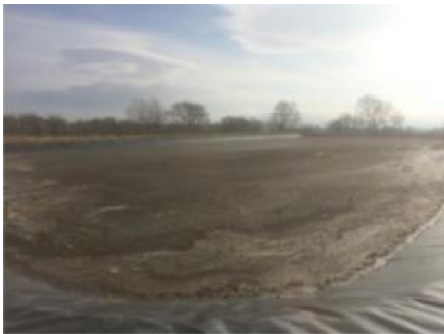
1 week's water savings after completion
