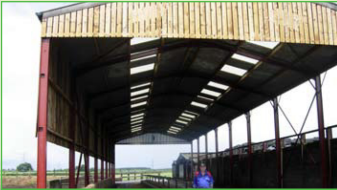
Part CSF funded roof over feed area
