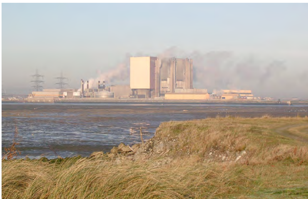
Large-scale industrial installations such as the nuclear power station at Hartlepool are juxtaposed with internationally designated inter-tidal habitats.
