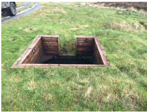
Figure 21 Example of Existing Butts
