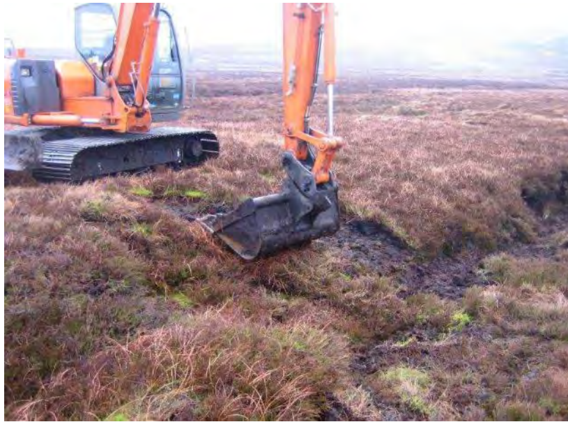
Figure 6: Typical reprofiled gulley edge
