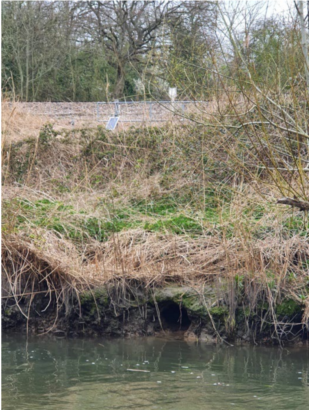
Figure 18. Burrowing activity in close proximity (<15m from tracks) to railway along Great Stour. Photo credit: Beaver Trust
