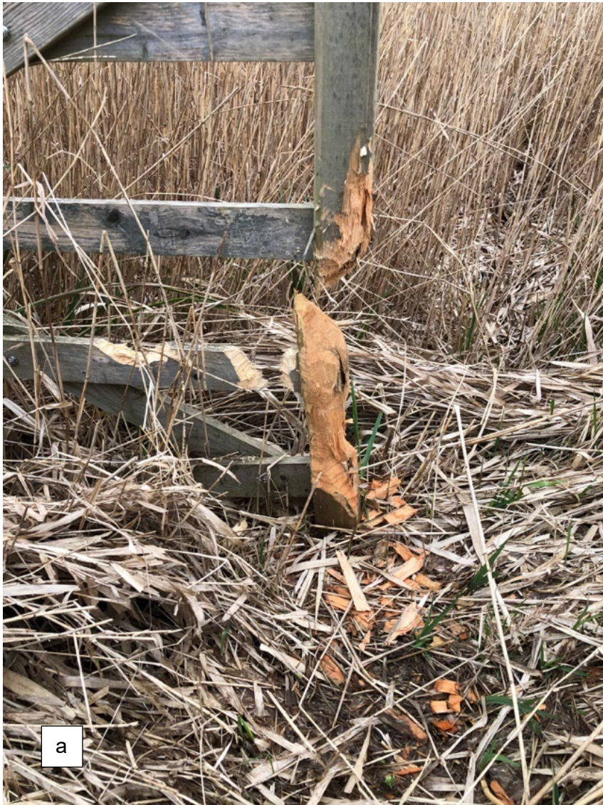
Figures 24 a and b. Gnawed gates at Stodmarsh NNR. Photos credit: Beaver Trust
