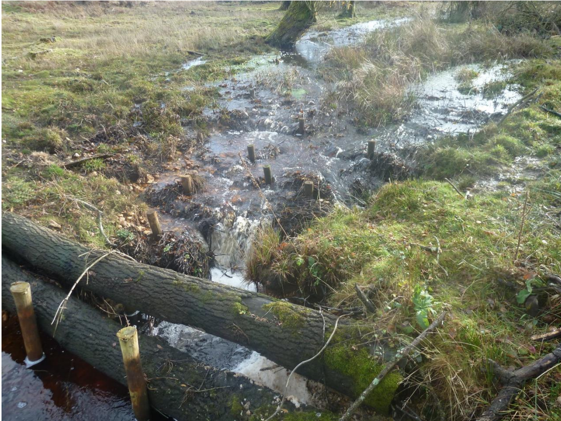
Figure 1-13: Pinned log and staked bail restoration
