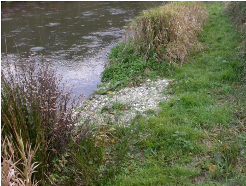
Fig. 13: Reinforced river banks at Upper Woodford (work undertaken in 2009)
