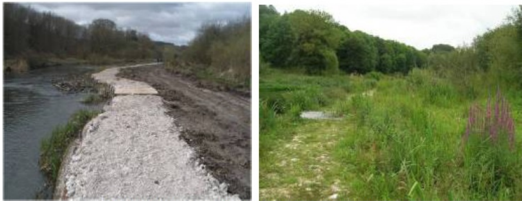
Reinstated access Feb 2009 and (right) in July 2009
