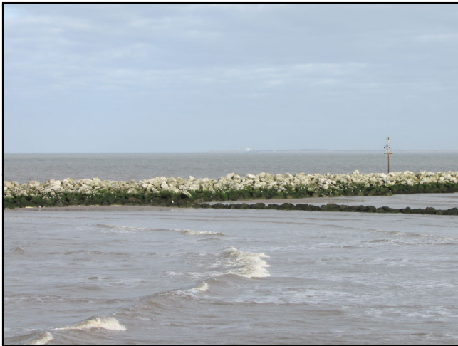
Photograph 3: View north, Leasowe. Offshore breakwater used as high-tide roost.
