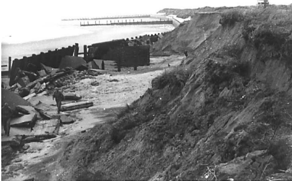
**Figure 19 January 1960: Dune erosion behind collapsed revetment along the Neck (from Phillips 1962)**
