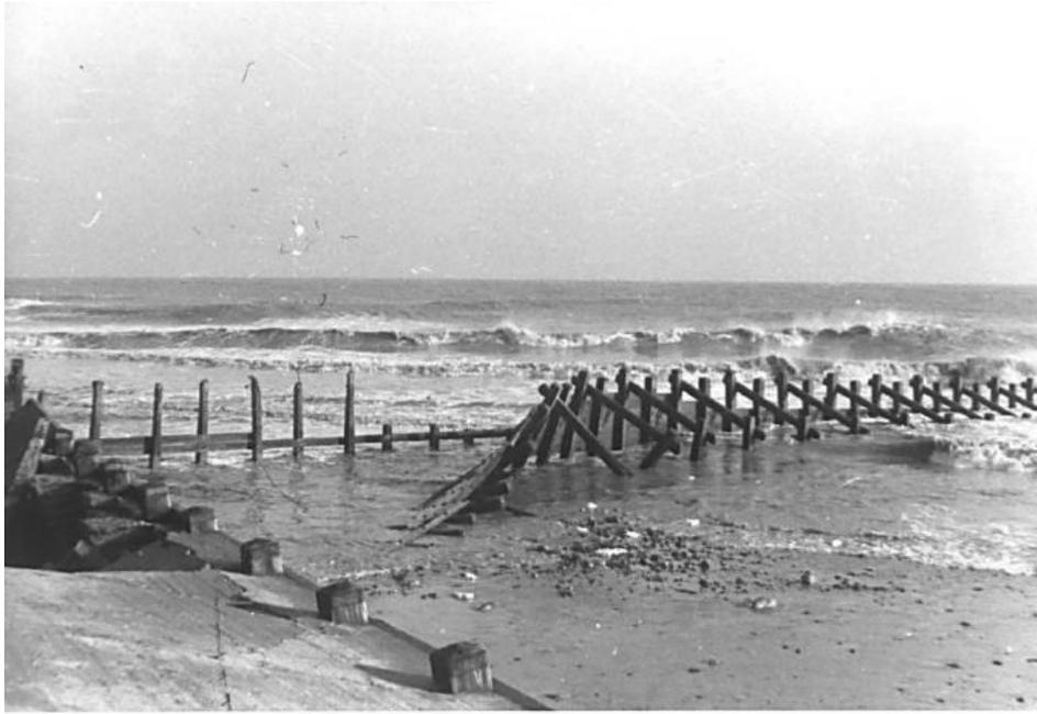
**Figure 17 January 1960: Broken groyne and collapsed revetment along the Neck (from Phillips 1962)**
