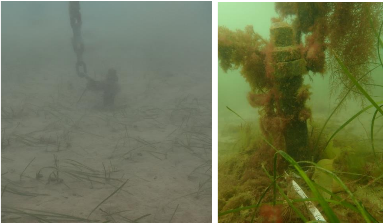
Photo: Helical screw anchor in place on boat mooring in Cawsand bay (Mark Parry, Ocean Conservation Trust (left image) and Natural England dive unit (right image))
