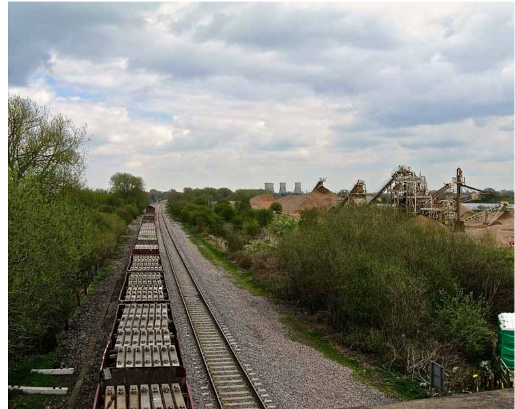
Gravel workings and train line near Willington looking towards the redundant cooling towers of the former power station site.
