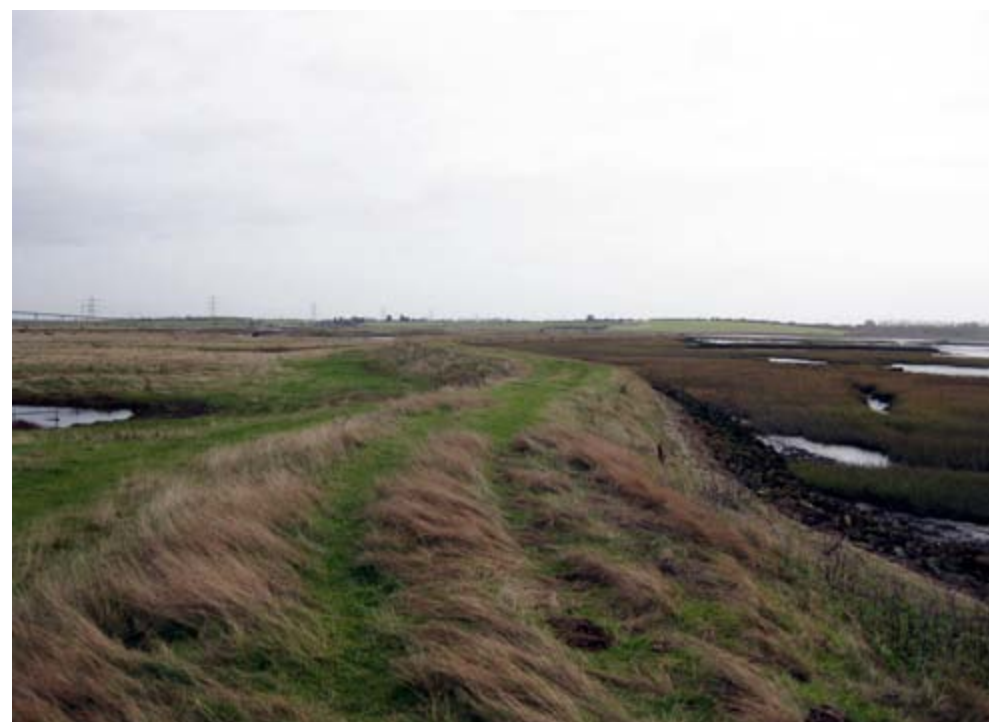
Sea wall flood defences in the Swale, with saltmarsh in front and grazing marsh behind.
