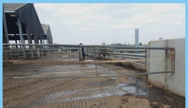
Channel constructed alongside existing lagoon to transfer slurry to reception pit.
