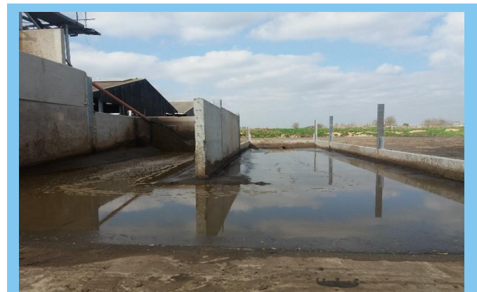
Sand sedimentation lanes flowing through 250mm pipe to lagoon in the background.
